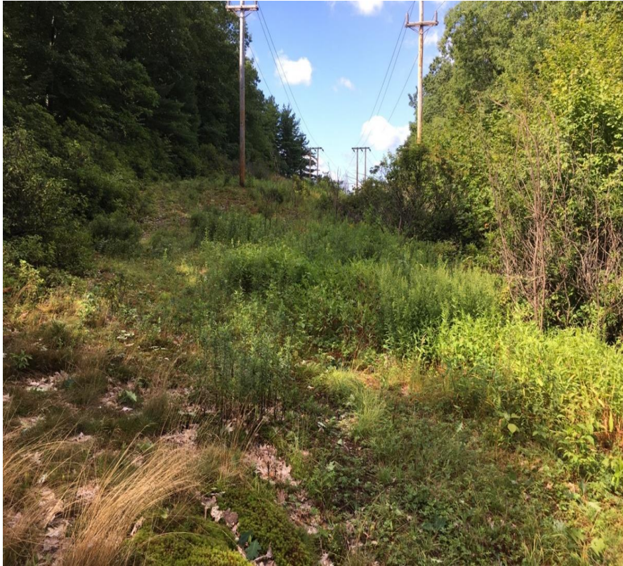
Example of Tap Line Structures.
